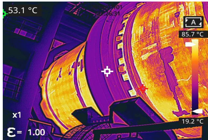
Figure 9.4 Defect Detecting of Refractory Material in Rotary Kiln
